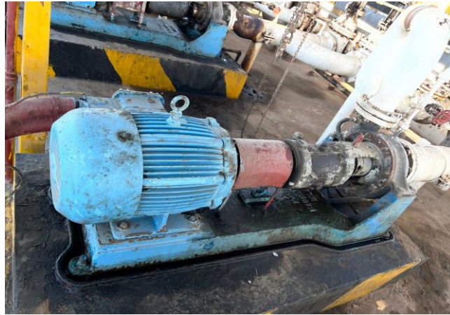
Figure (2): Foundation of a Centrifugal Pump at Al-Brega Company.
