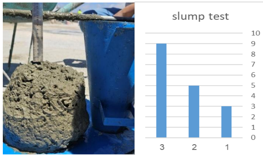
Figure 4. Slump test of the fresh concrete
