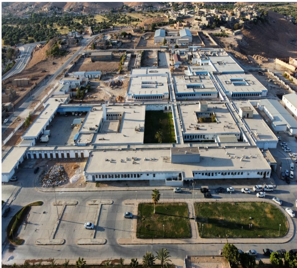
Figure 1: Bani Walid Hospital, Libya
